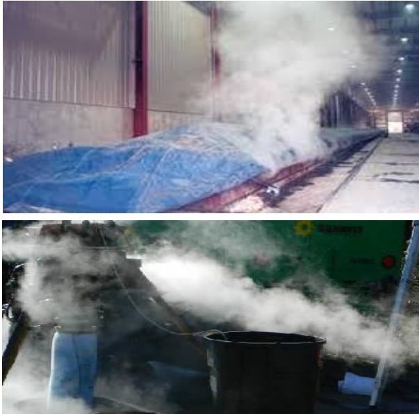
Fig.: Steam Curing
