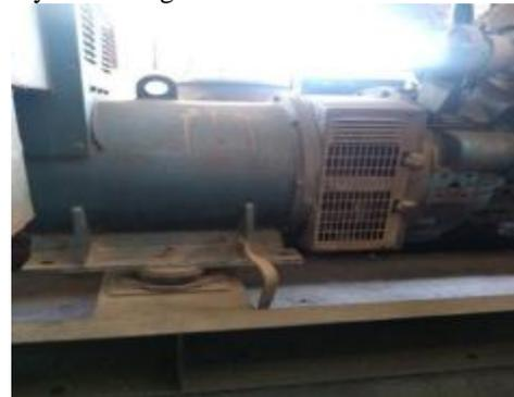
Fig 9: Dg Set -Body Earthing
