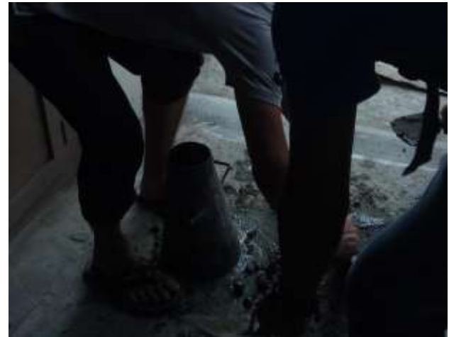
Figure 7: Conducting Slump cone test
