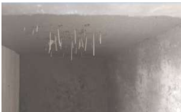
Fig: Inserting the optical fibers
