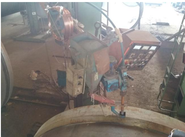
Figure 1: Image during submerged arc welding of tower
