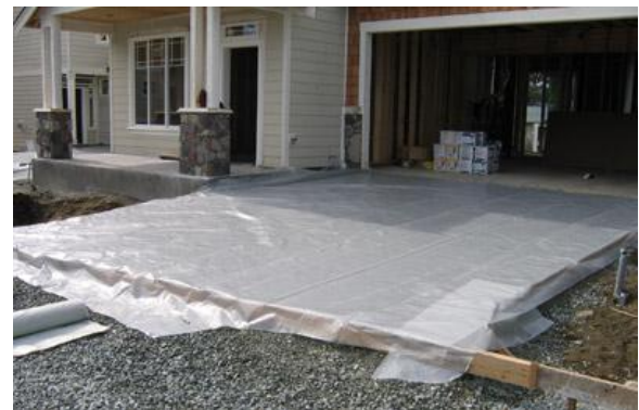
Figure 4: Concrete curing using plastic wrap.
