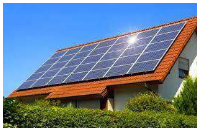
Fig. 4 Rooftop Building Management System
