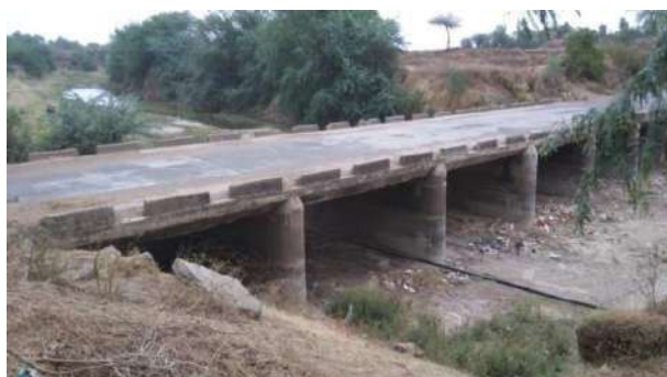
Figure 9: Lack of Lighting and Safety Signage
