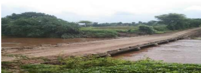
Figure 1: High Level Causeway at Naved-Darapur Road
