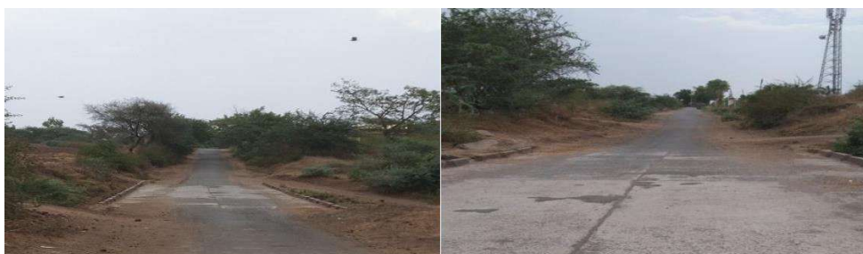
Figure 7: High Slope Road Connecting the Bridge
