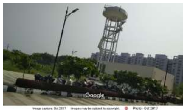
Fig. 1 – Constructed water tank at IGNOU, Lucknow (Courtesy - Google maps)
