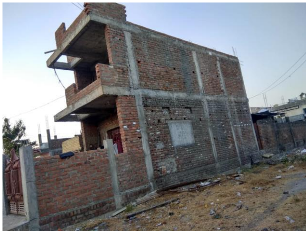
Fig. 10- Old masonry building (Amravati, India)
