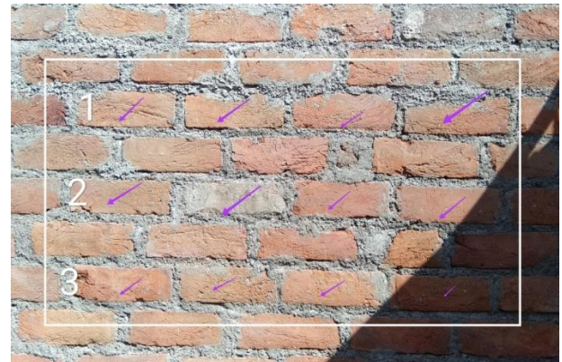
Fig. 11- Front view of wall
