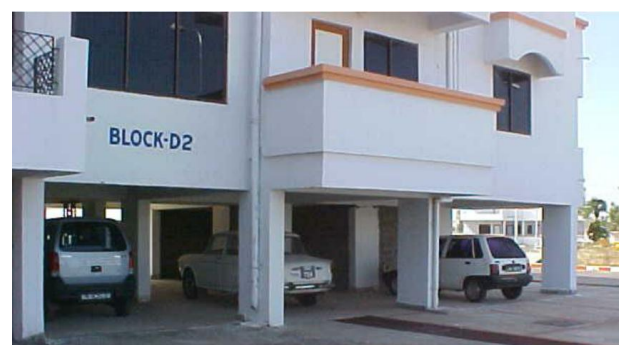
Fig.1 - Open ground Storey of the building
